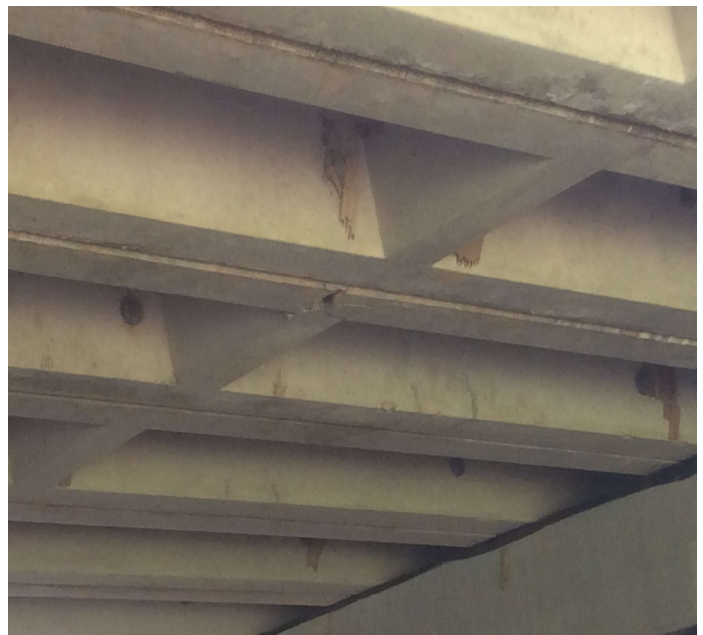
PHOTO 2 Description Span 4 unit 5 small spall on bottom of channel leg.
