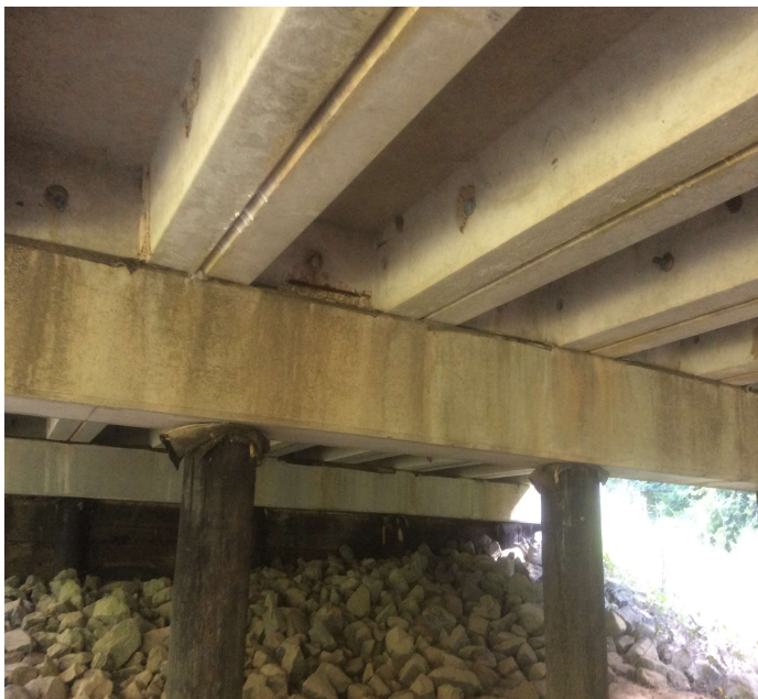
PHOTO 1 Description Span 2 at bent 2 unit 6 small spall in diaphragm . Common bent 3 span 3 unit 3
