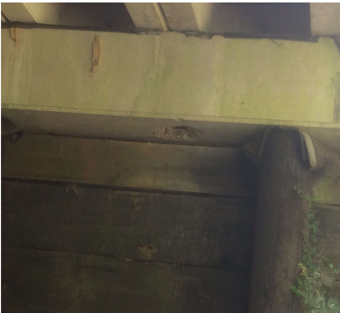
PHOTO 1 Description Bent 5 bottom of cap between pile 4 & 5 small spall with exposed rebar.
